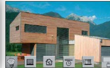
A family home in low energy standard in Innsbruck (Austria)
