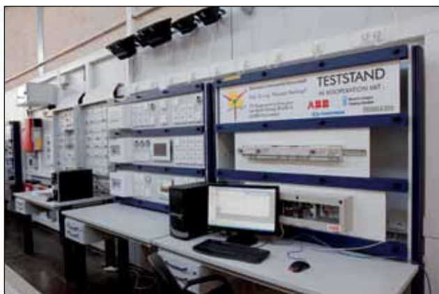
On the KNX test stand, the students can configure and test functions with ETS as they would do in a house
