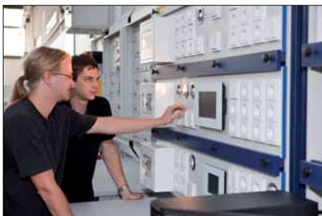
The touch screens on the test stands indicate whether the load management functions are as required
