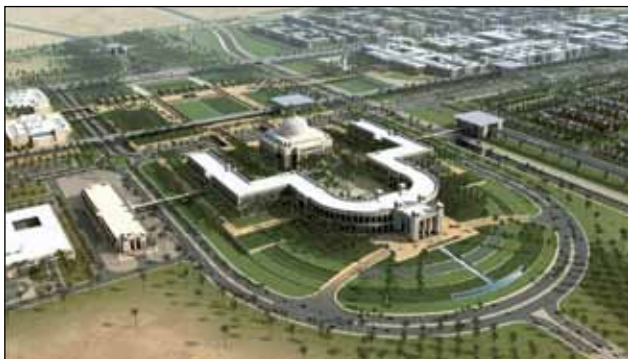
The campus of the Princess Noura University for Women is impressive due to its size, architecture, comprehensive teaching programme, social facilities – and due to its highly modern building system technology
